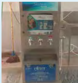
Installation of RO Unit at Government School
